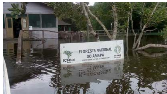
The flooding in the area.
